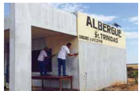
Maintenance work at the Holy Trinity Home
